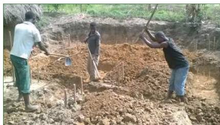
Workers laying the foundation
