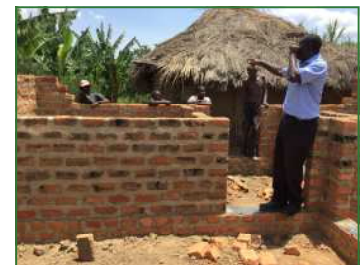
The Trust Administrator monitoring the progress of the house
