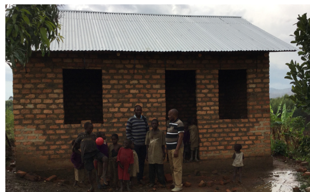
George Kakongozo's new house under construction by BMCT
